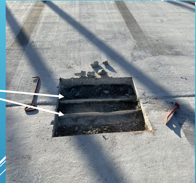
Floor Joint Opening
