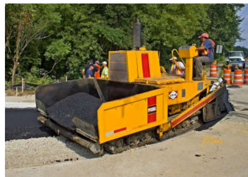
Hot mix asphalt (HMA) paver will place the new road surface.
